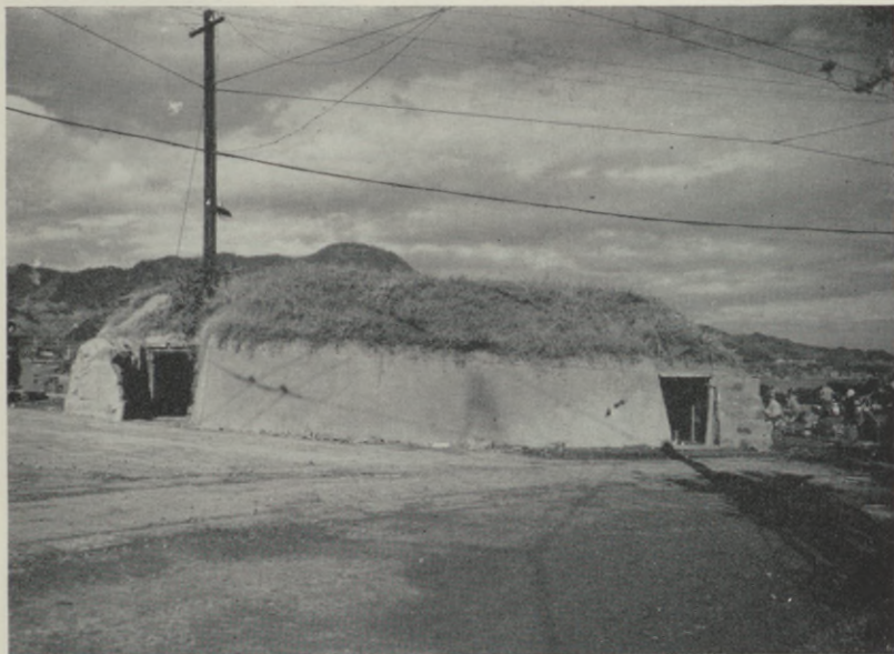
Photo 30. Concrete square shelter built for and by the navy personnel located at Nagasaki port. Concrete thickness at the base approximately 4 feet, tapered to 3 feet on top. Roof is of 2 feet by 2 feet planks, reinforced by approximately 1 foot of concrete and 4 feet of dirt at the thickest point.
